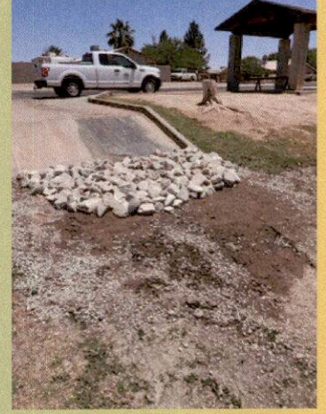
Spillway was reconfigured so it would have better drainage
