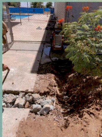
Installed a 2" pipe conduit to pass fiber optic line from Youth Center to the Pool
