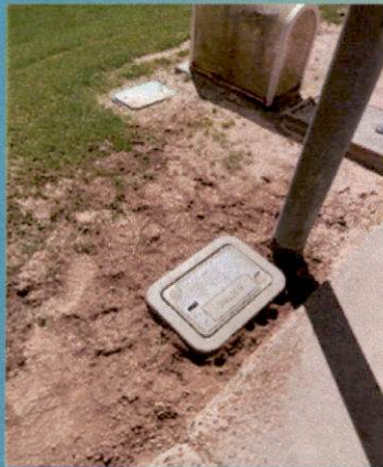
Electric boxes were installed to replace damaged boxes
